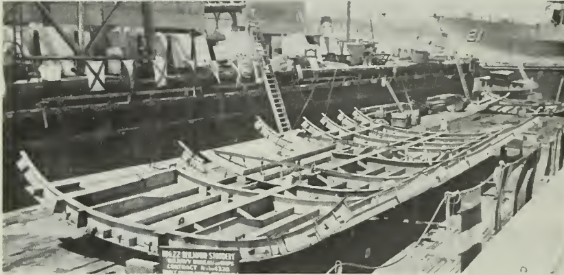
(3) Crane lowers section of bottom
